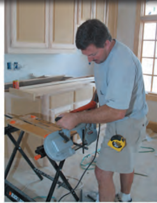
2. Cut baluster to length.
