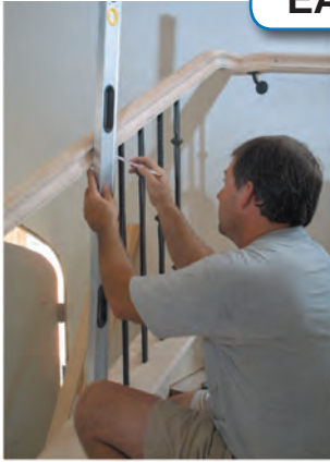
1. Check for plumb of baluster length and placement.
