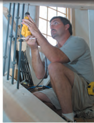
3. Cut round hole in bottom of handrail for baluster.
