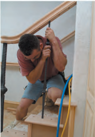
7. Install baluster into epoxy filled holes and press in for tight fit.
