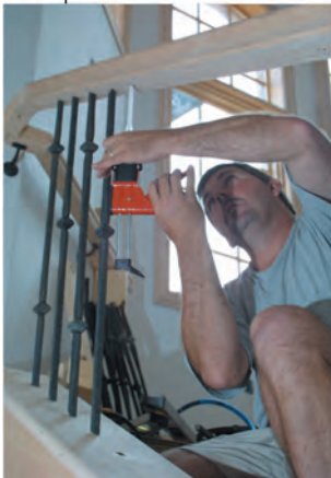
5. Apply epoxy in hole for baluster on top.
